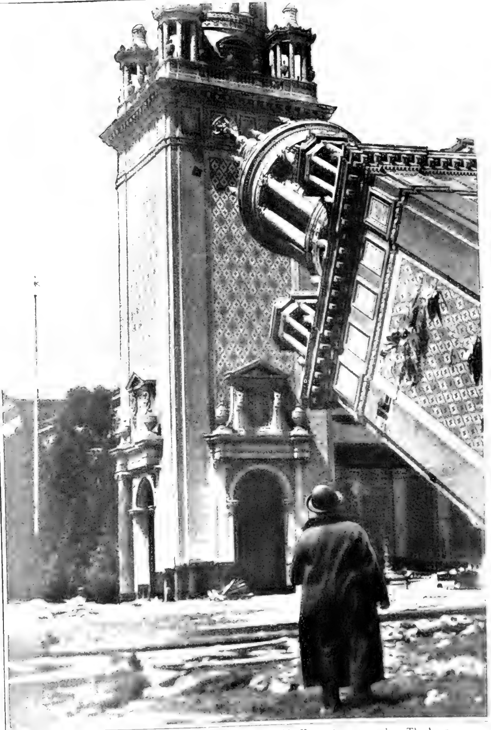
Wrecking the Italian Towers at the Panama-Pacific Exposition grounds. The base
